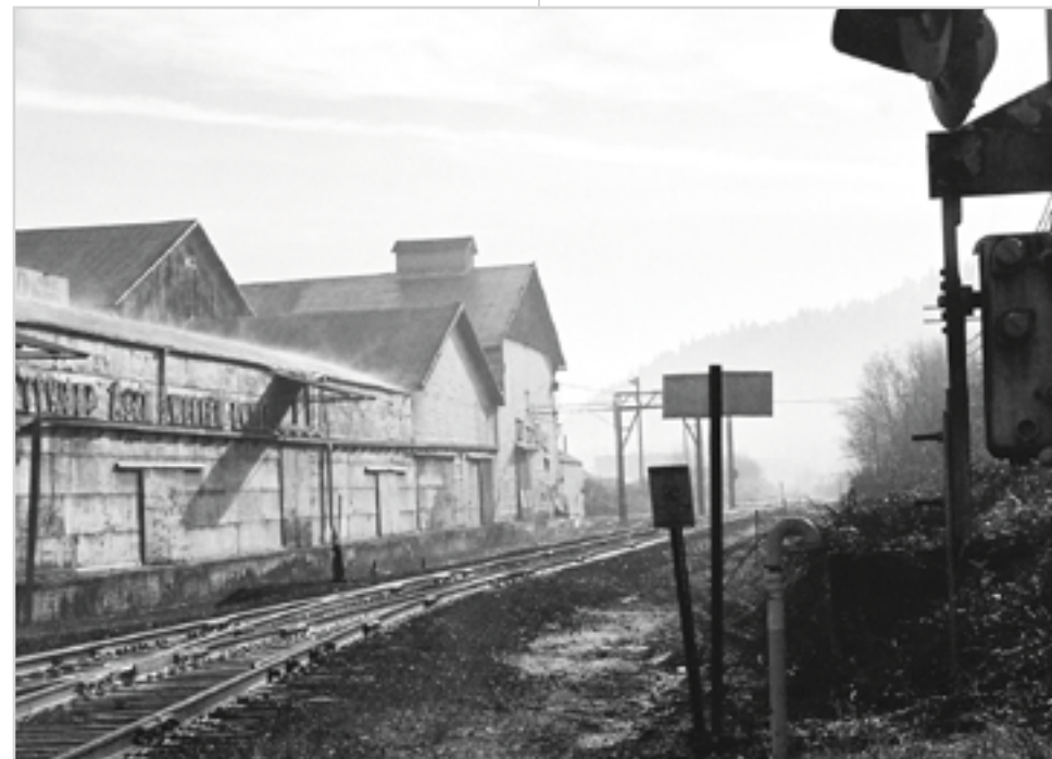
■ Living on the right side of the tracks? Will the Linnton Plywood factory be the next Pearl District?
